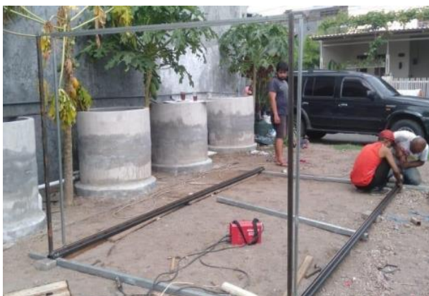
Figure 8. Welding of frame components (T-joints)
